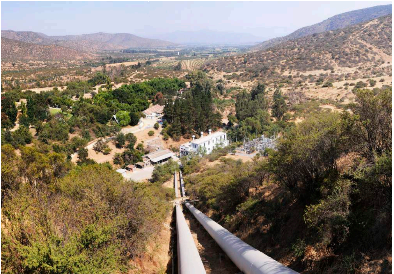
Power Station Carena
