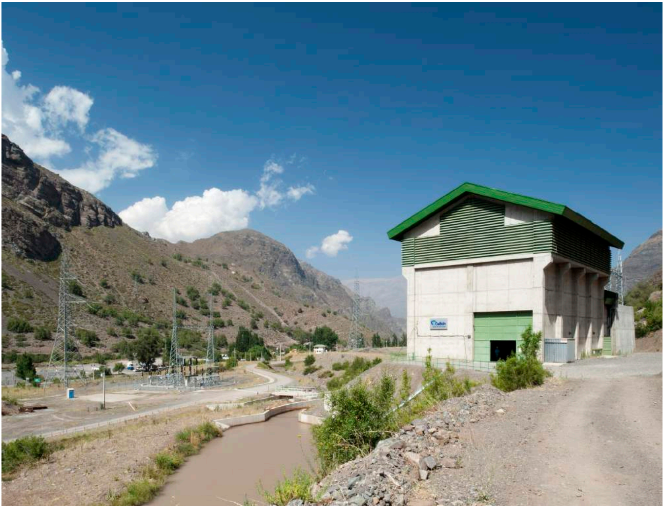
Hornitos Power Plant
