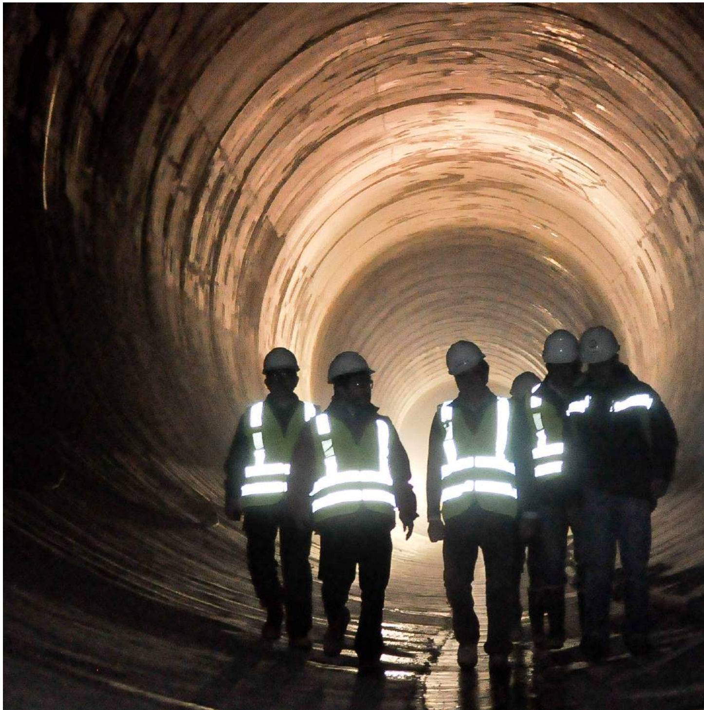
Power Station Angostura
