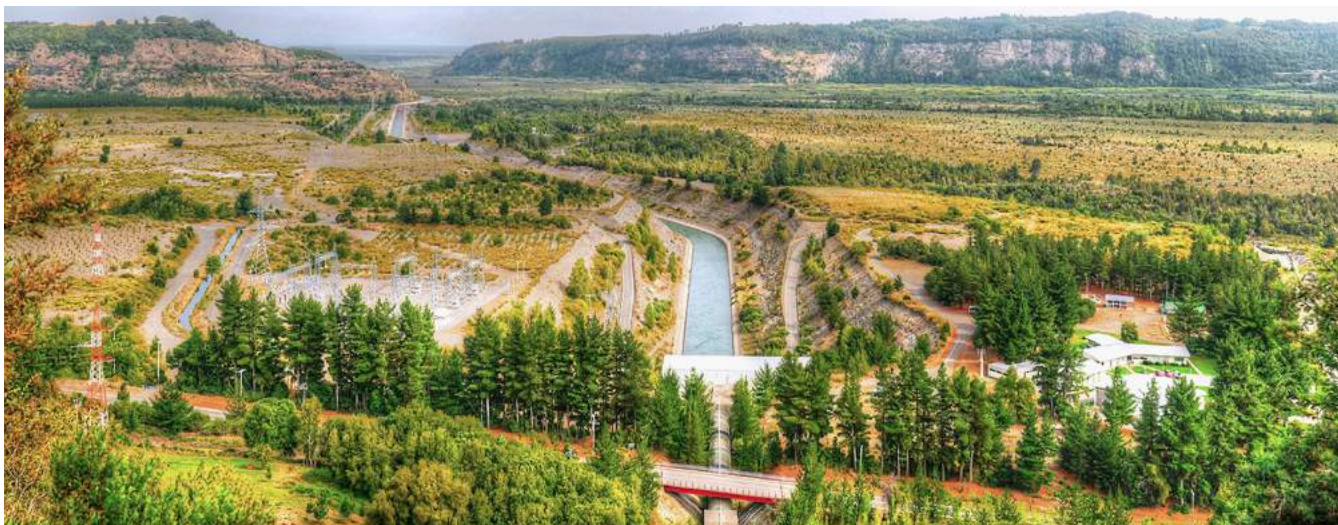
Power Station Rucúe
