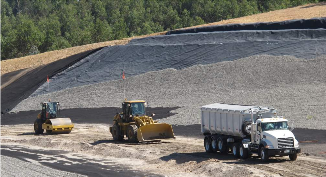
Contractors Santa María Complex
