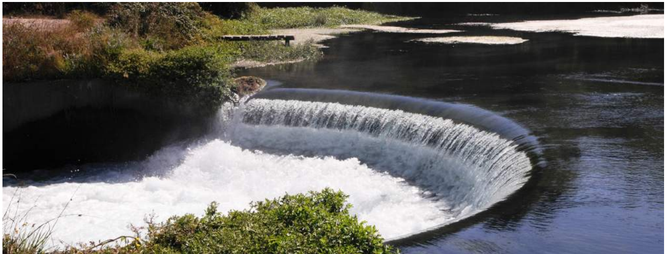
Colbún Power PLant
