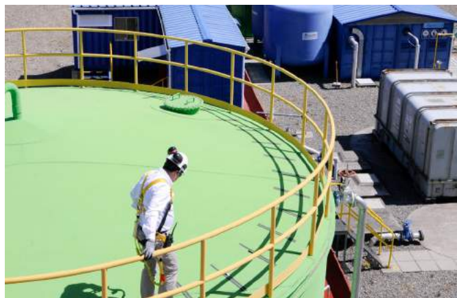
Antilhue Power Plant
