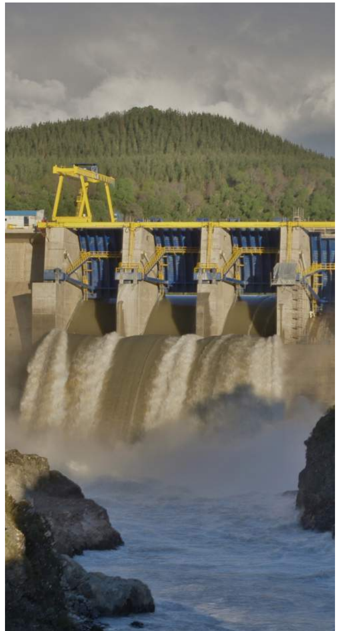
Angostura Power Plant
