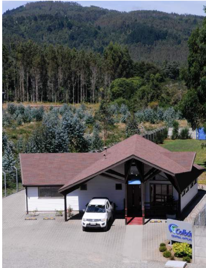
Antilhue Power Plant
