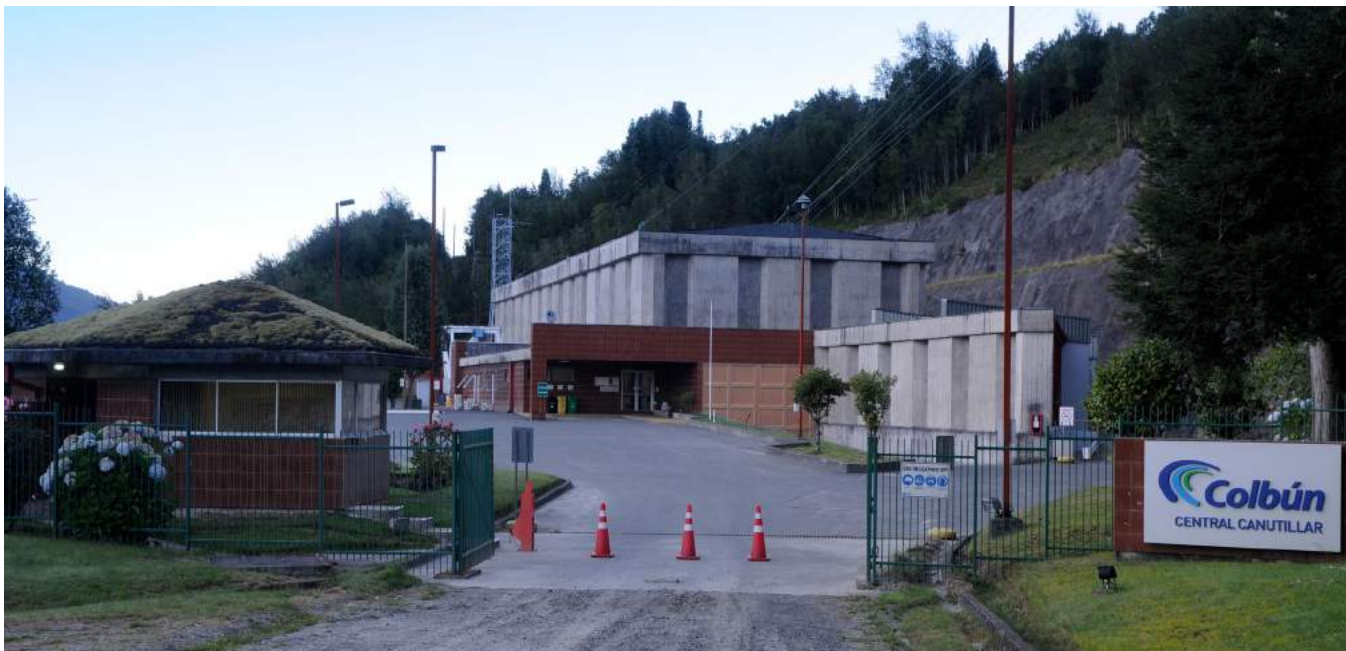
Power Station Canutillar
