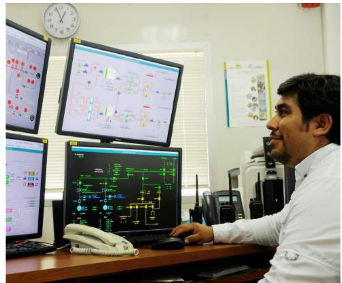
Operation center, Colbún S.A.
