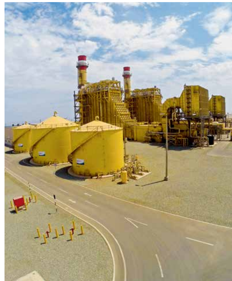
FENIX PERU POWER PLANT
