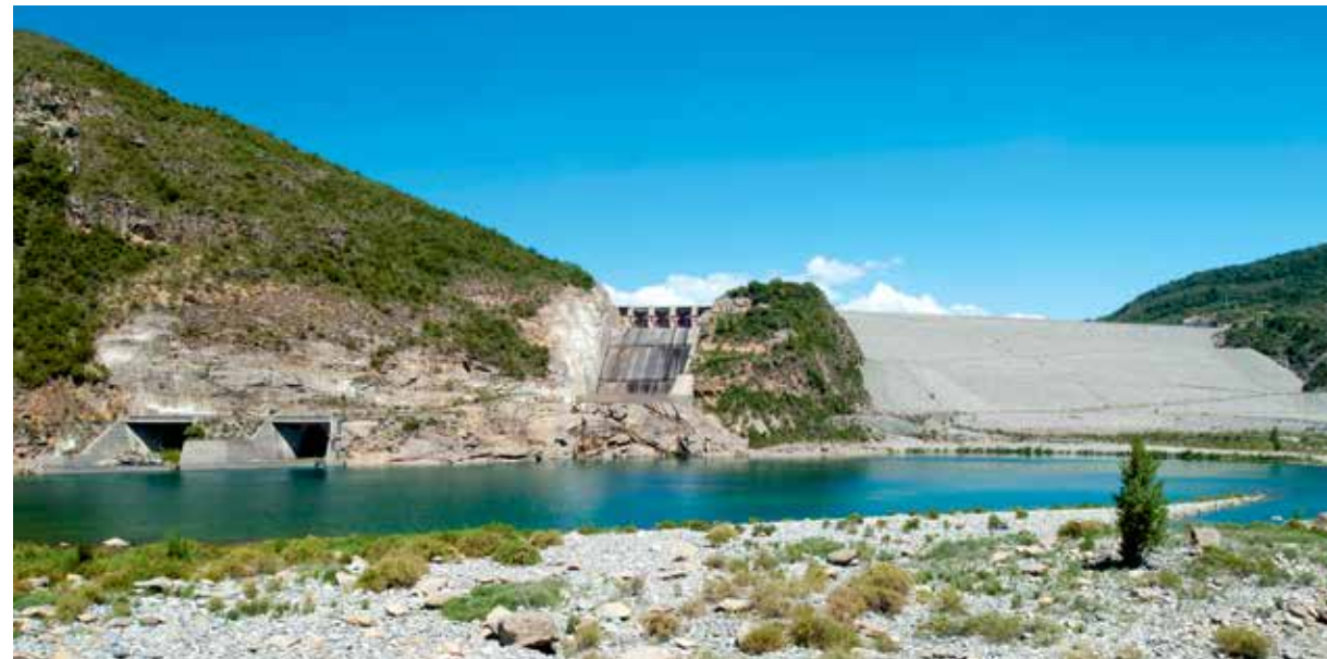
COLBÚN POWER PLANT
