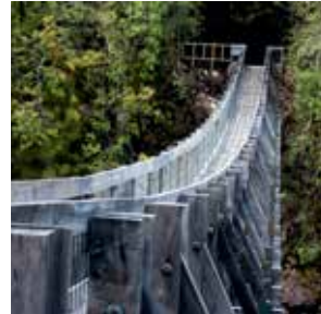
Suspension Bridge Canutillar Power Plant
