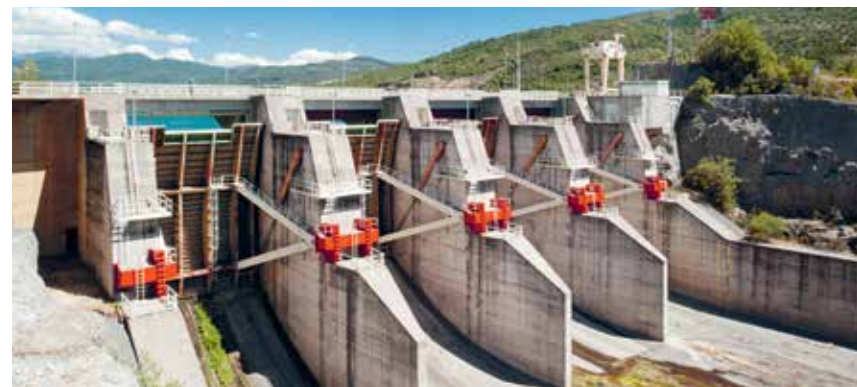
COLBÚN POWER PLANT
